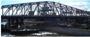
2005 –145th Street Bridge The 1<sup>st</sup> bridge built at the Port of Coeymans and delivered by barge to its permanent location in front of Yankee Stadium.
